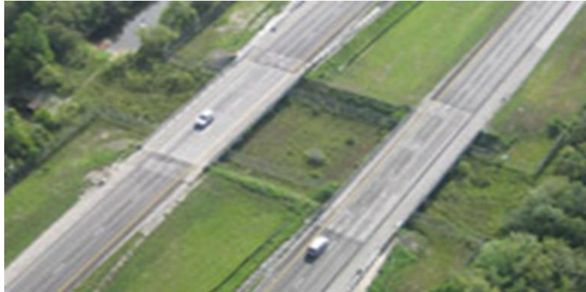
Cougar underpass beneath I-75 in Florida. Photo credit: Florida Fish and Wildlife Conservation Commission.
